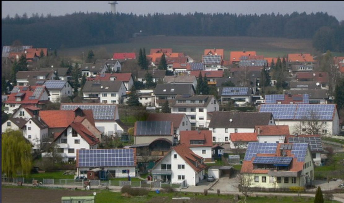
Rooftop Solar in Germany
