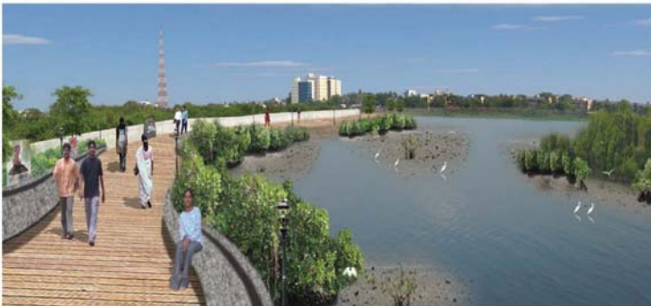
After transformation: Edges of the creek restored with mangroves and mudflats, sewage inflows stopped, encroachments removed and water front walkway established.
