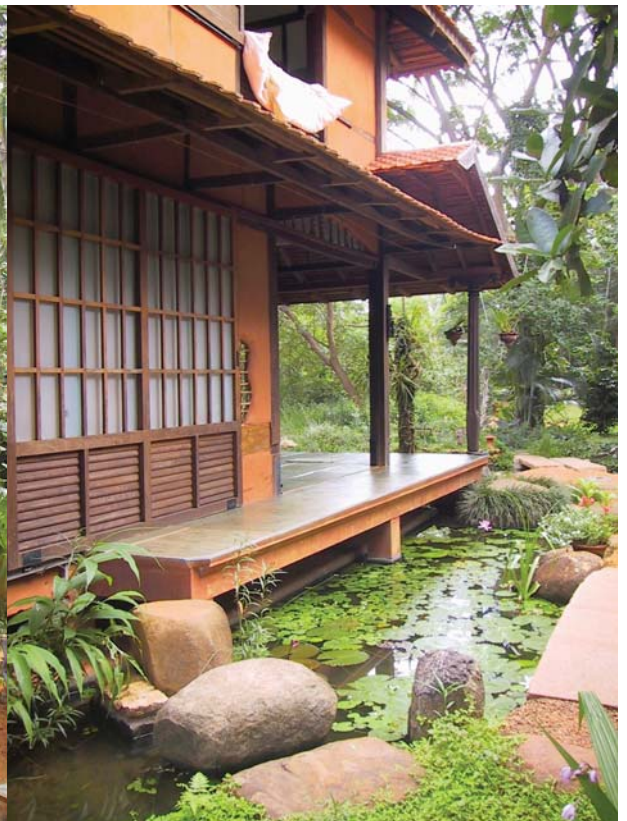
Wattle & daub with wooden shingles
