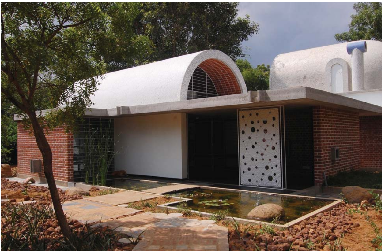
Domes & Vaults with brick
