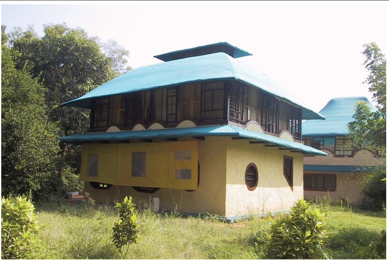
Light weight roofing
