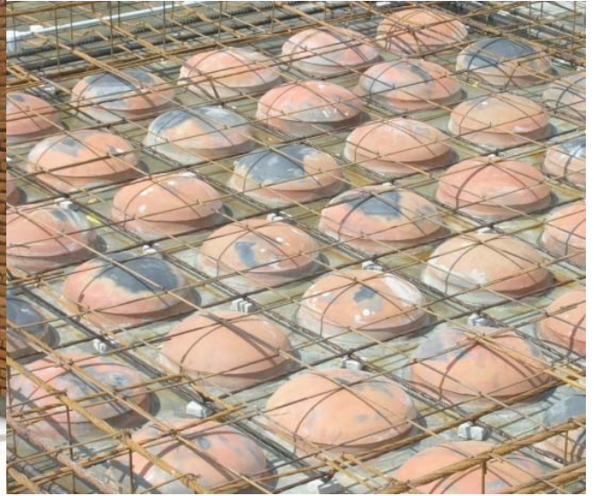
Filler slab with terracotta pots
