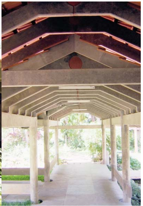
Precast rafters & tiled roof
