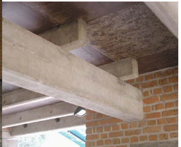
Flat roof with precast beams and stones
