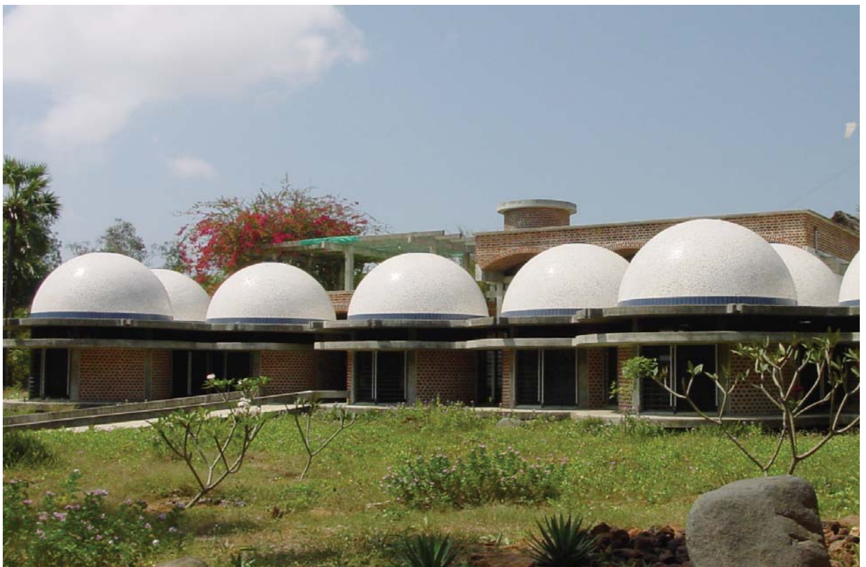
Domes & Vaults with brick
