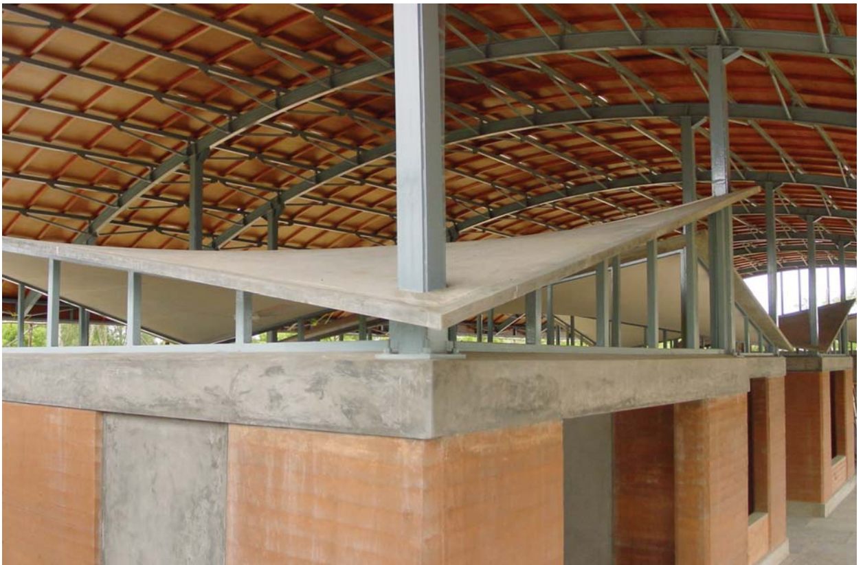
Light weight roofing
