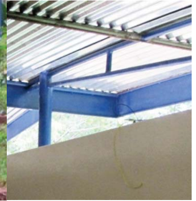
Light weight roofing
