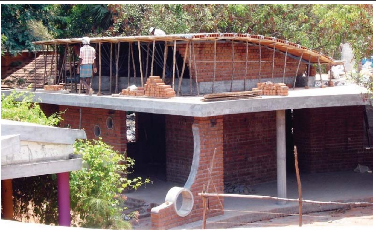
Roofing with terracotta hollow blocks
