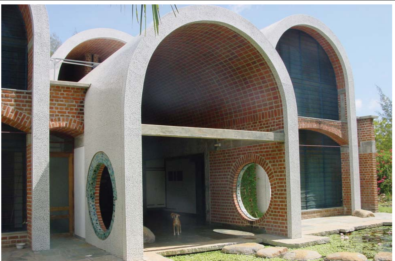
Domes & Vaults with brick
