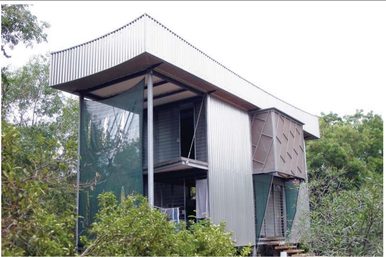
Light weight roofing
