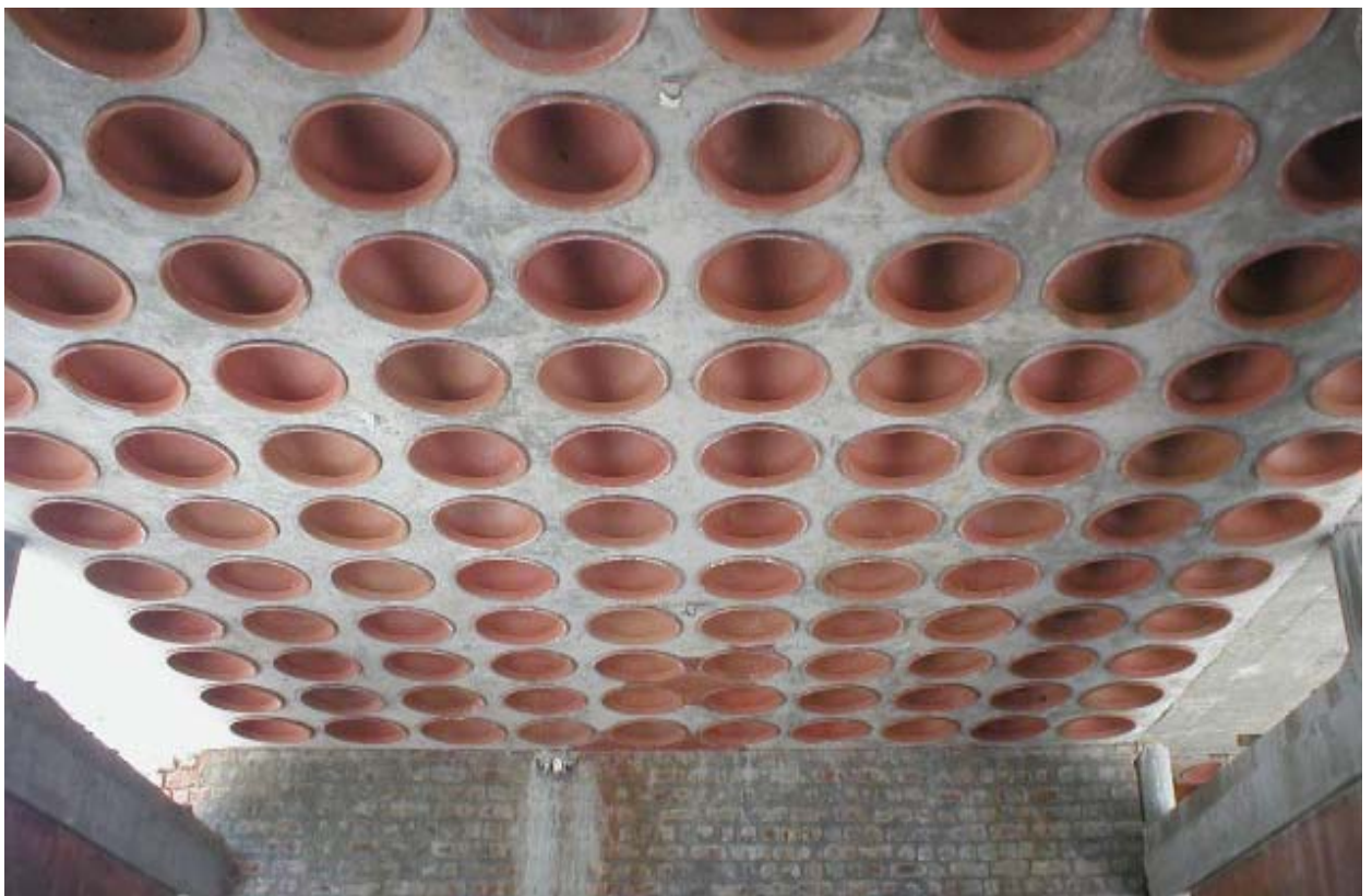
Filler slab with terracotta pots
