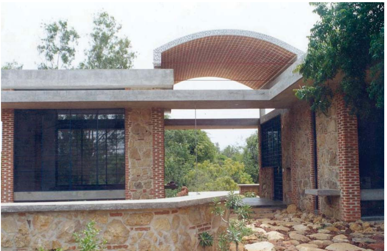
Load bearing limestone walls
