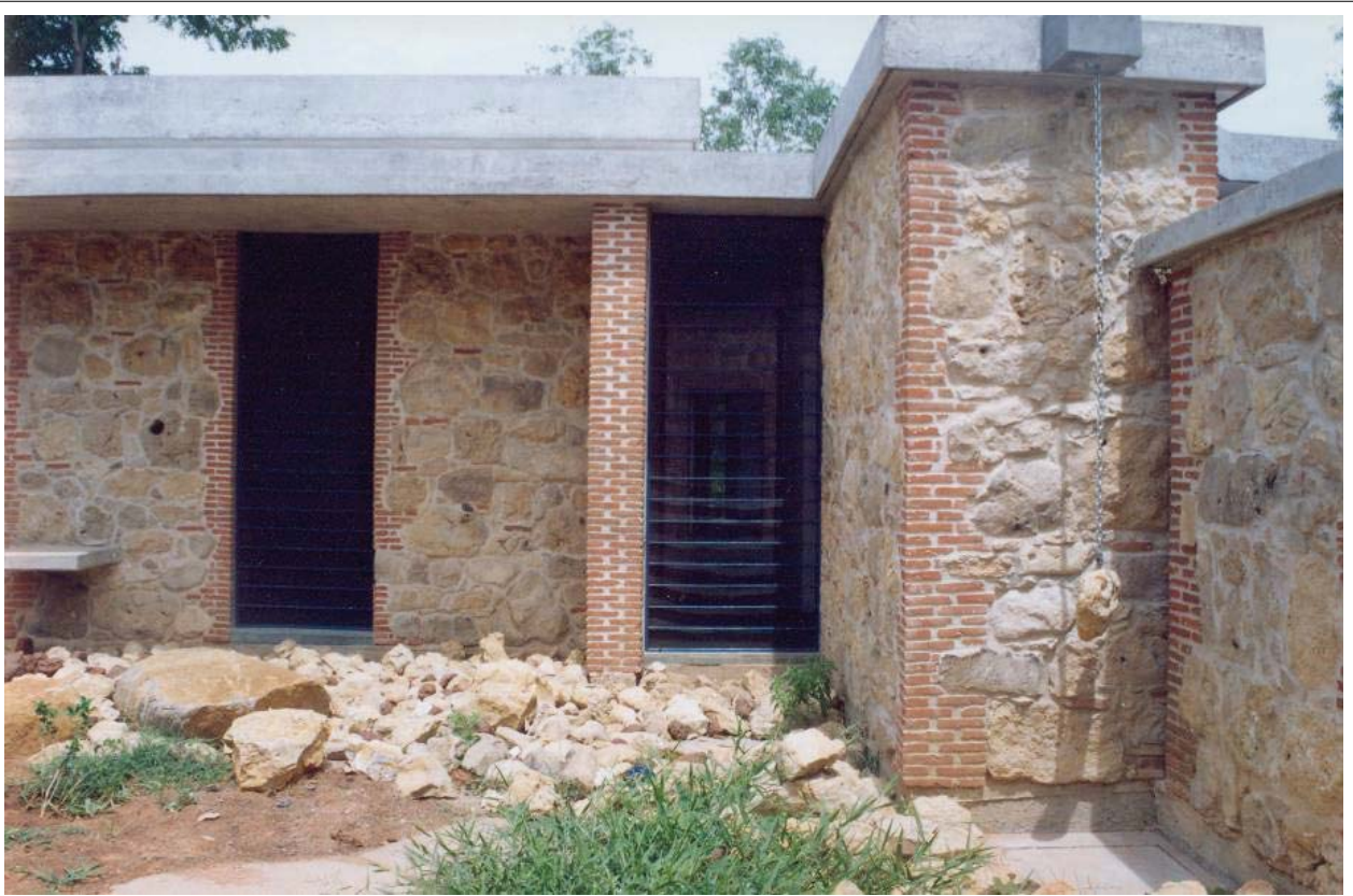
Load bearing limestone walls
