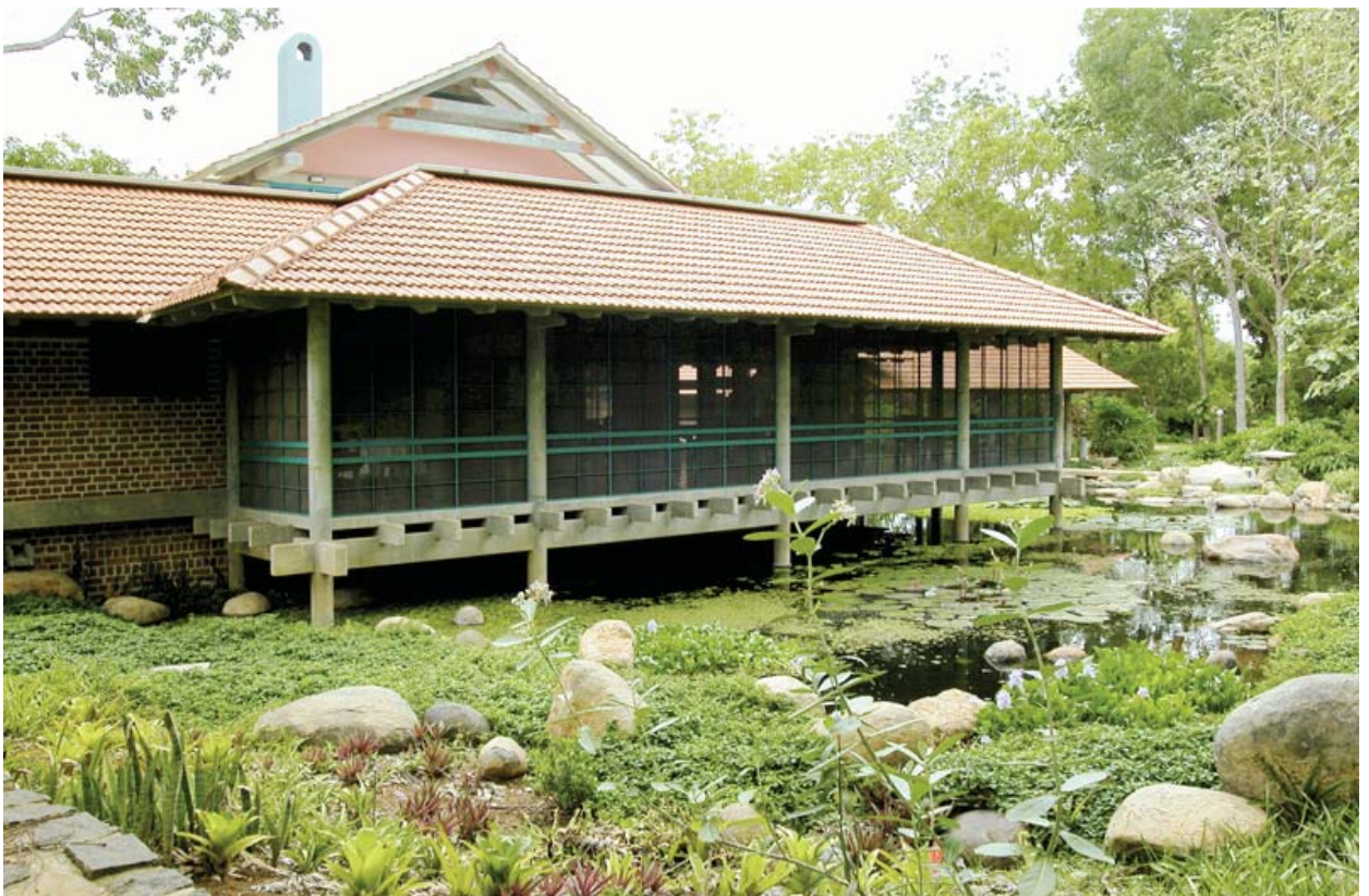
Precast rafters & tiled roof
