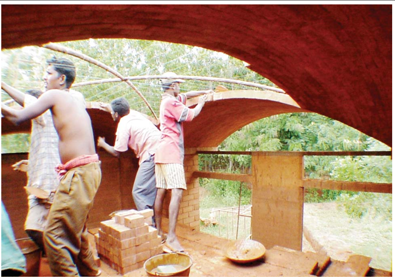
Building a groined dome with the Nubian technique
