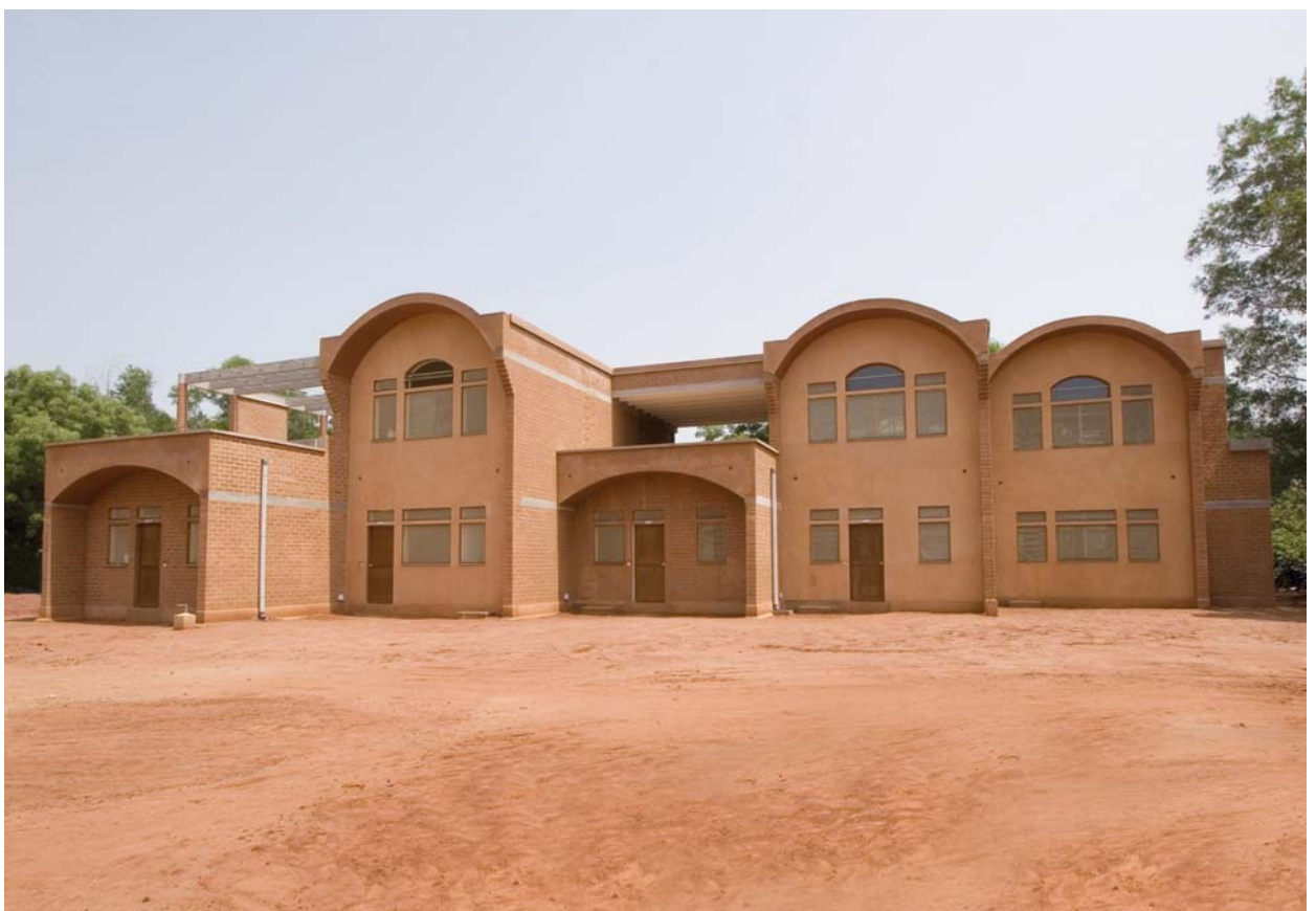
Realization - 5 Apartments completed
