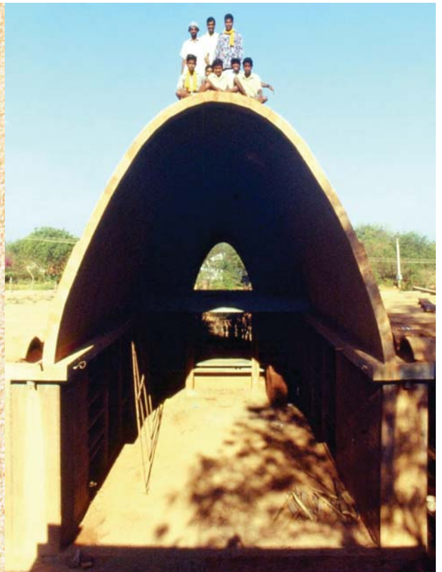
Building an Egyptian shaped vault with the Nubian technique, 5 m span, 9 m long Completed in 12 days with 4 masons
