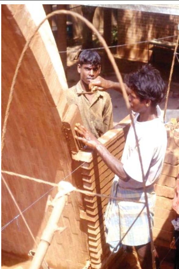
Building a lunette, 1.2m span with the Free Spanning technique
