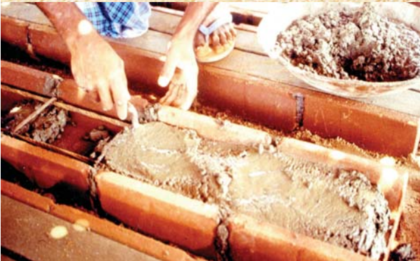
Composite lintel single height
