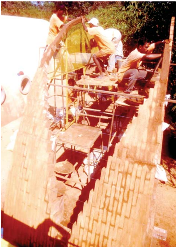
Building an Egyptian shaped vault with the Nubian technique, 5 m span, 9 m long Completed in 12 days with 4 masons
