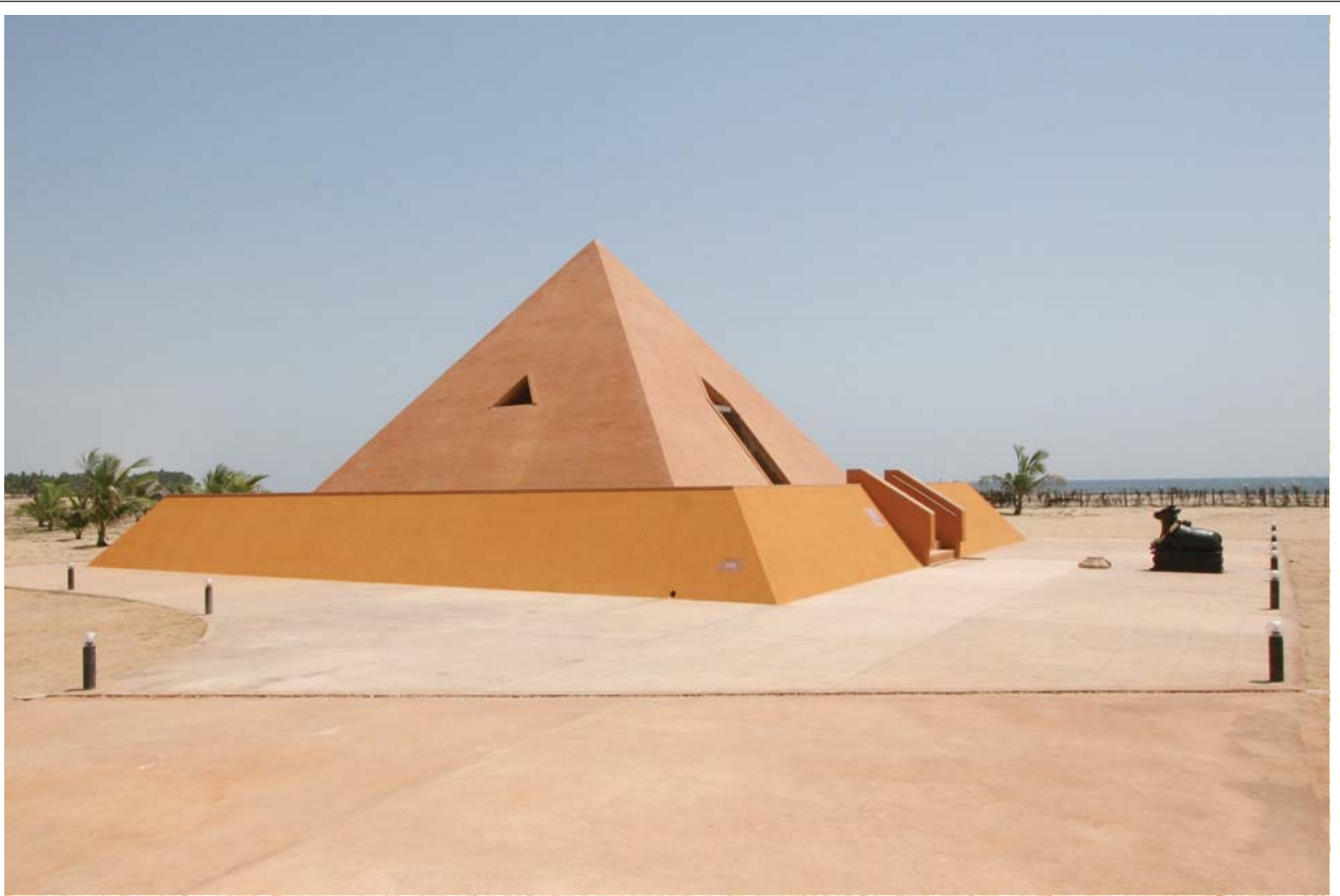
Sri Karneshwar Nataraja Temple near Auroville Pointed cloister dome 6 m span and pyramid, built in 6 months
