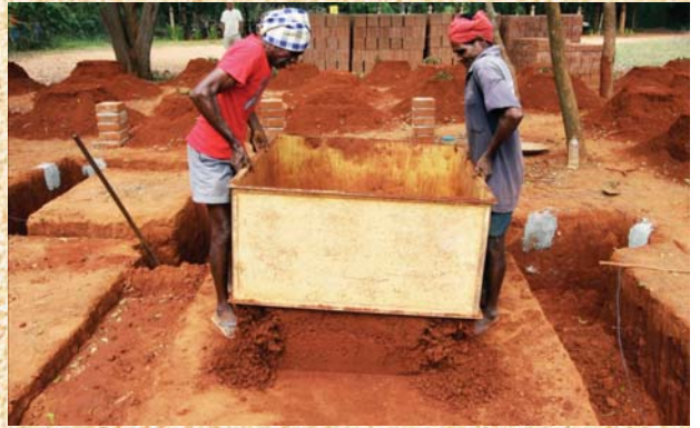
Lifting the frame
