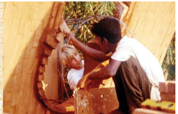
Building an Egyptian shaped vault with the Nubian technique, 5 m span, 9 m long Completed in 12 days with 4 masons
