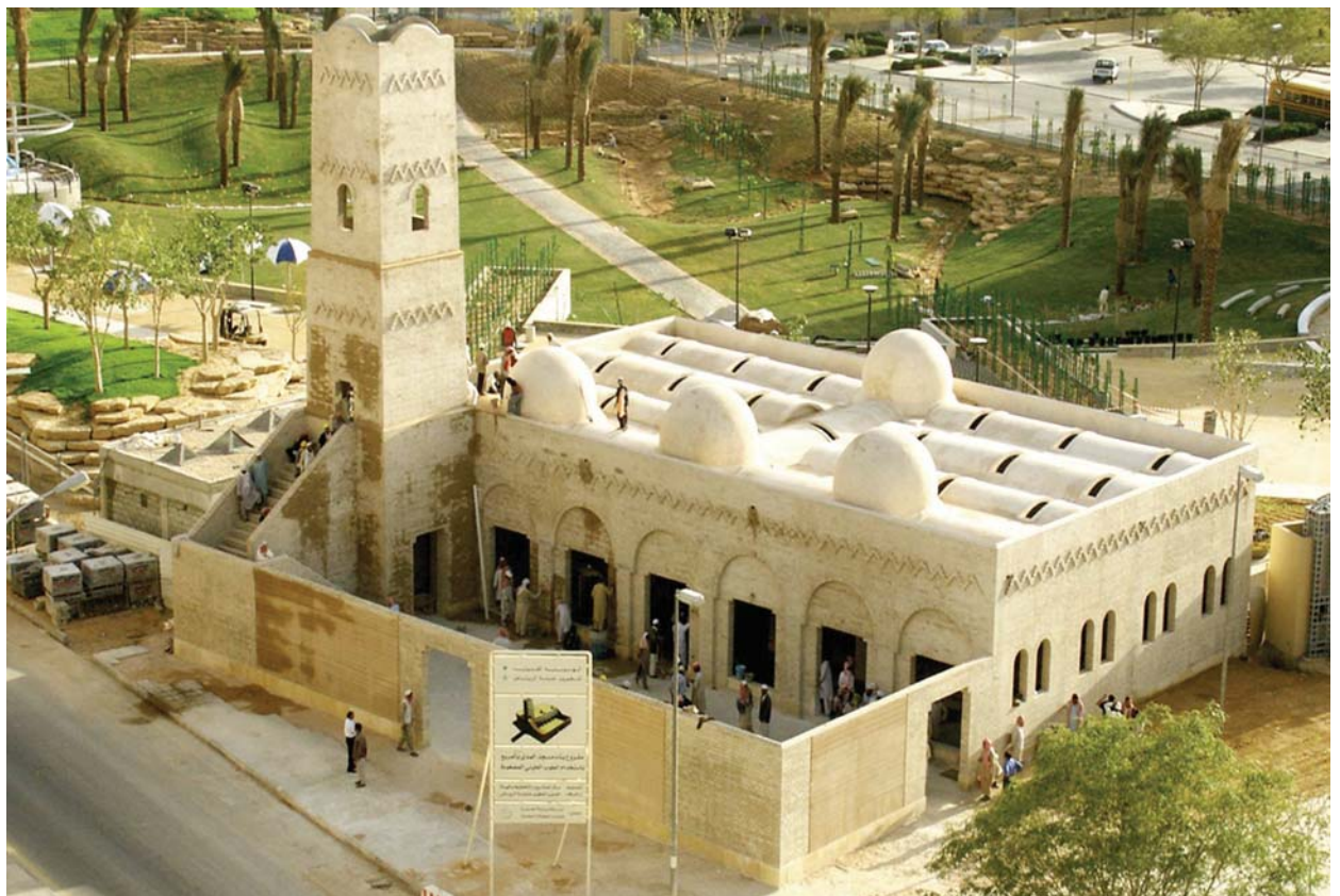
Al Medy Mosque built in the heart of Riyadh , 420 m 2 , 18.05 m high minaret Built in 7 weeks with ~ 75 unskilled masons and ~ 150 workers
