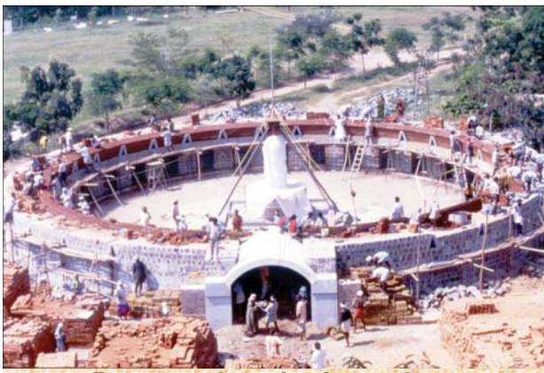
Dome and vault after 5 days
