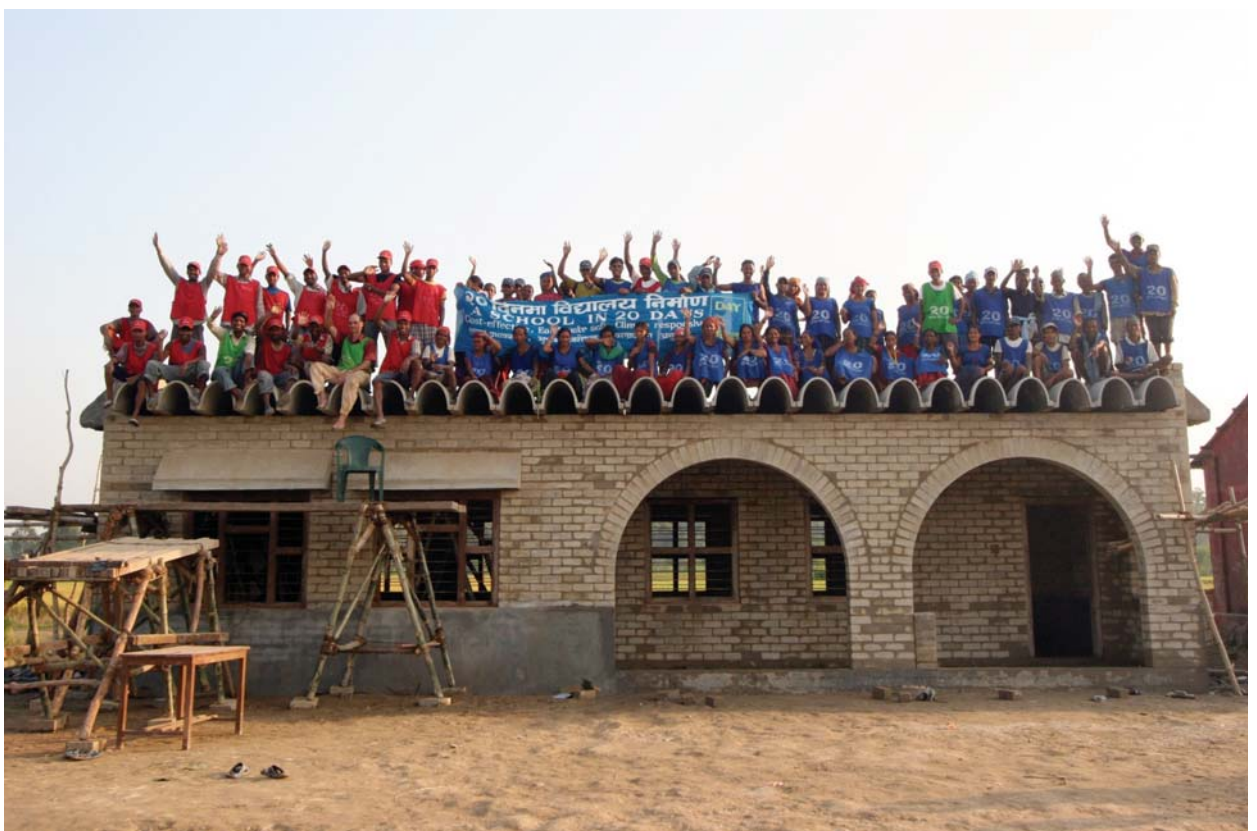
Nepal – Jantanagar school, built in 20 days Earthquake resistant, climate responsive – Built with community participation
