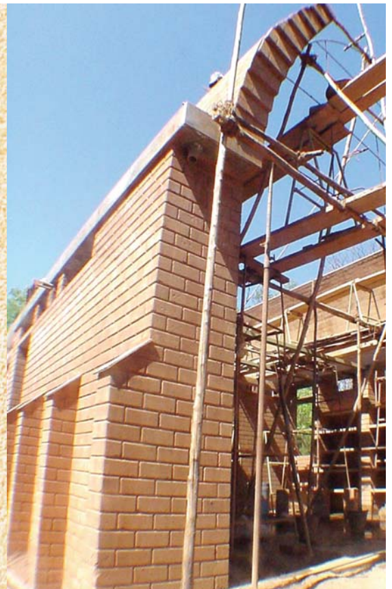
Building a semicircular vault with the Free Spanning technique - 6 m span, 11 m long
