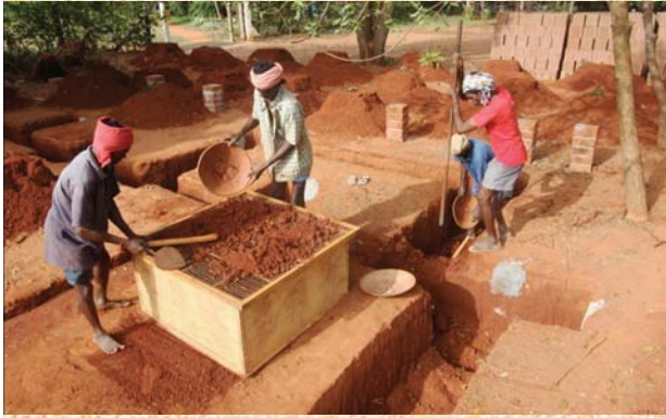
Digging the trench and filling the frame
