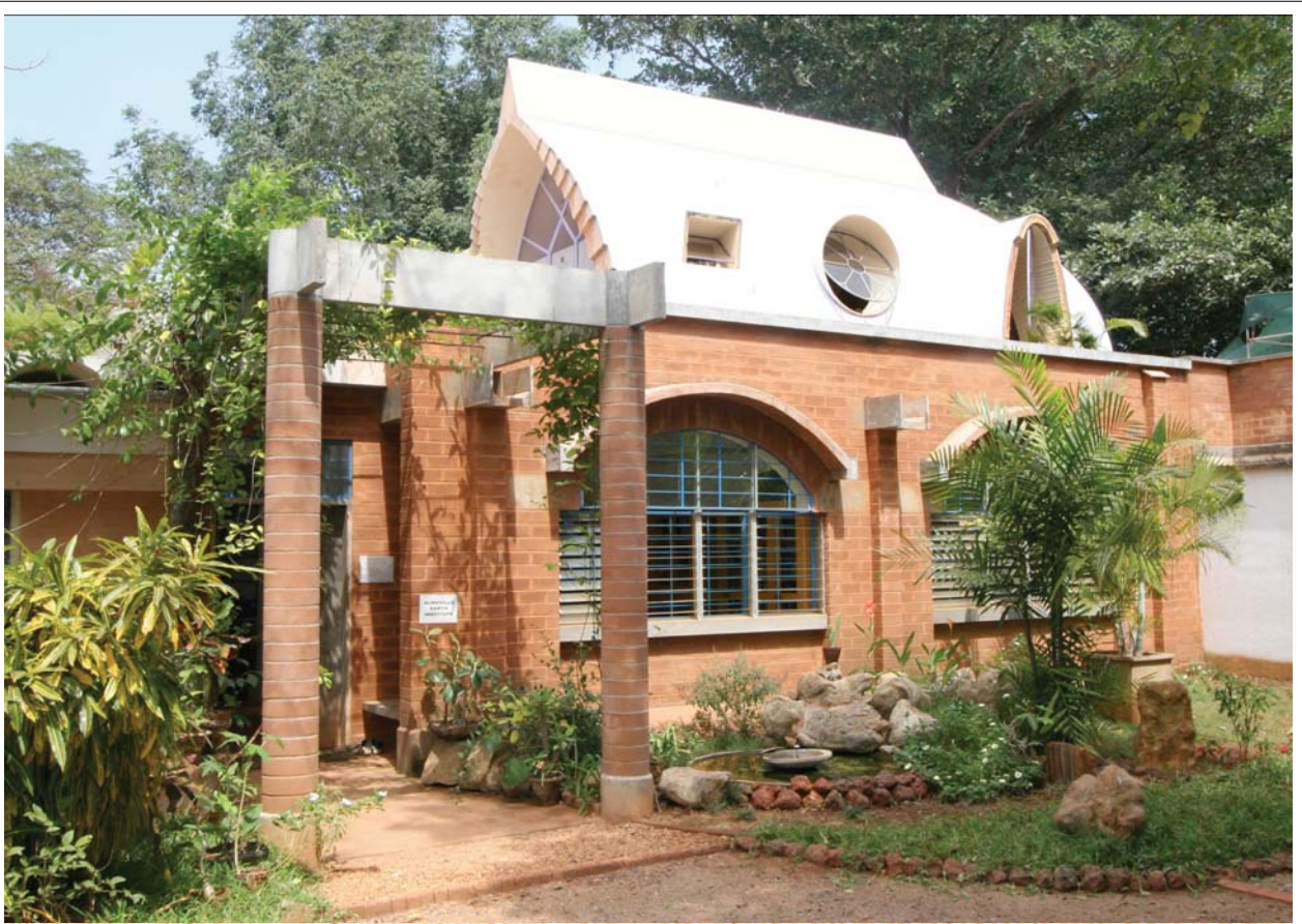
Office of the Auroville Earth Institute
