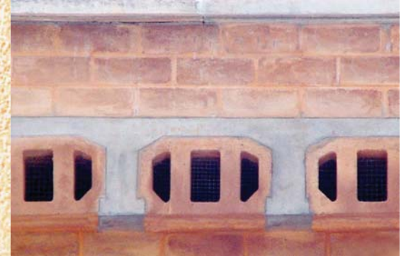
Hourdis blocks and T beams
