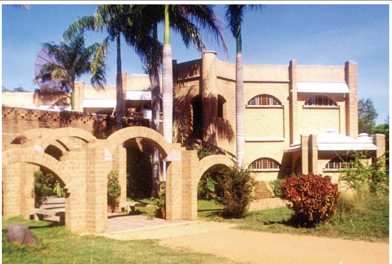
Visitors Centre, 1200 m 2 1992 Hassan Fathy International Award for Architecture for the Poor
