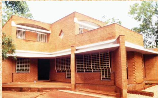
House at Dana community
