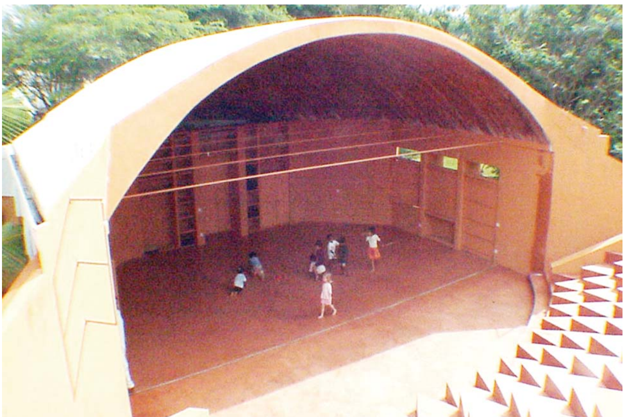
Deepanam School near Matrimandir - Stabilised rammed earth walls and CSEB vault 10.35 m span, 2.25 m rise
