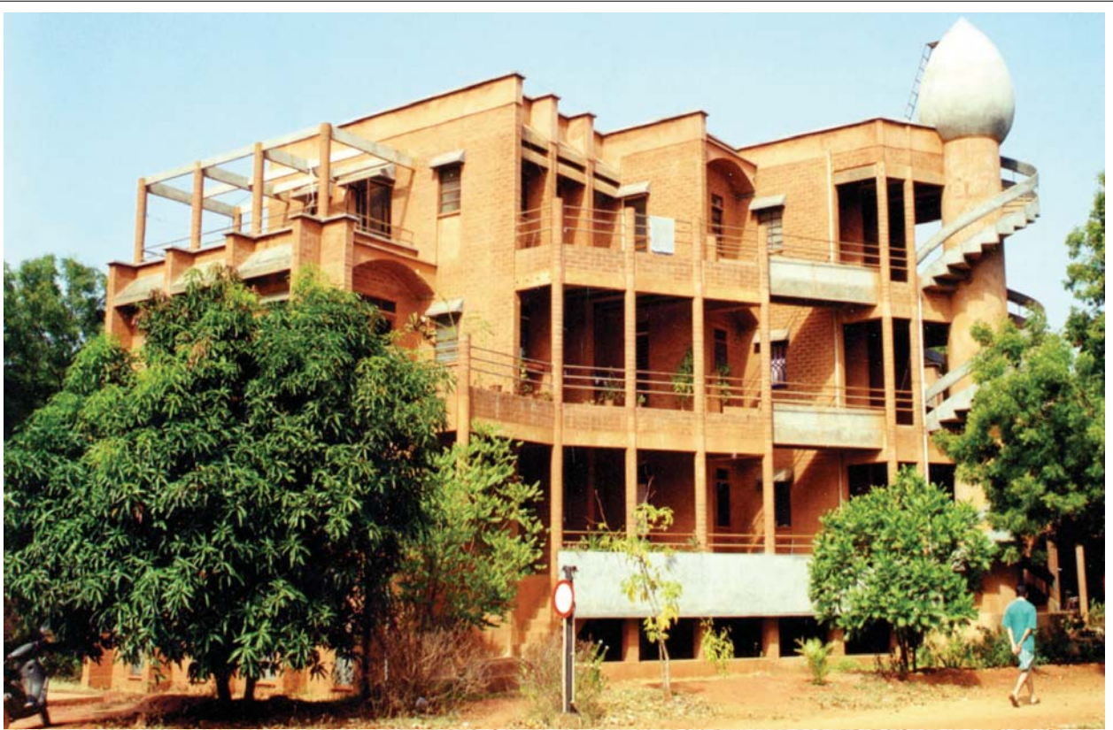
13 apartments on 4 floors at Vikas Community Vikas Community was a finalist for the “2000 World Habitat Award”
