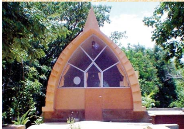
House at the Auroville Earth Institute, built with the Free Spanning Technique
