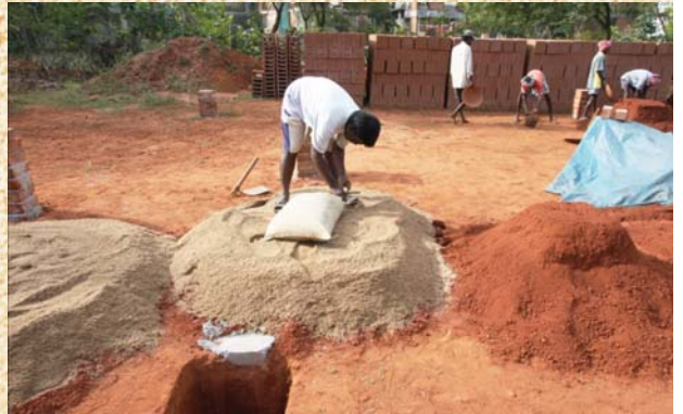
Adding 200 Litres of sand and 1 bag cement
