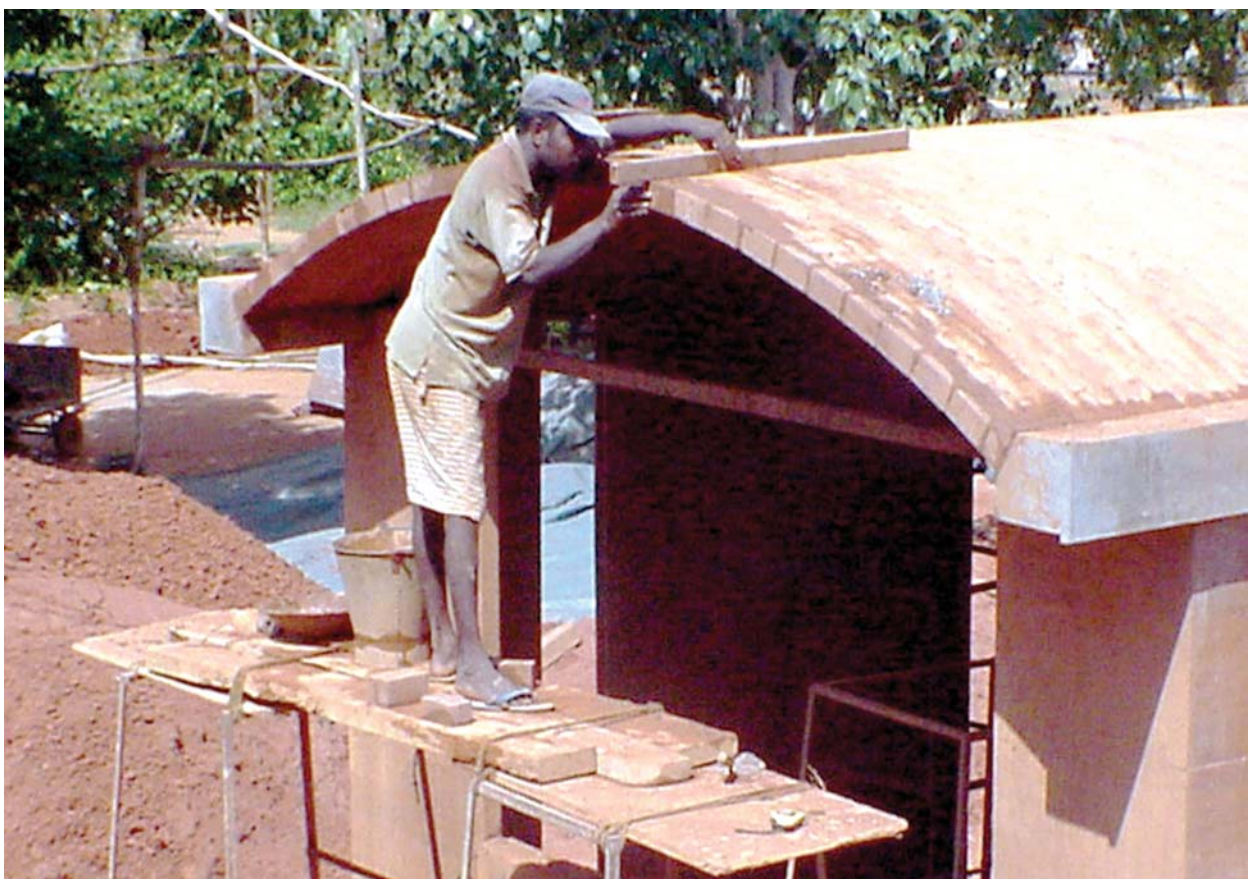
Building a segmental vault with the Nubian technique
