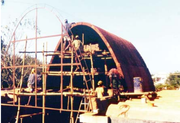
Building an Egyptian shaped vault with the Nubian technique, 5 m span, 9 m long Completed in 12 days with 4 masons
