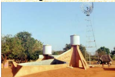
Half underground reservoir
