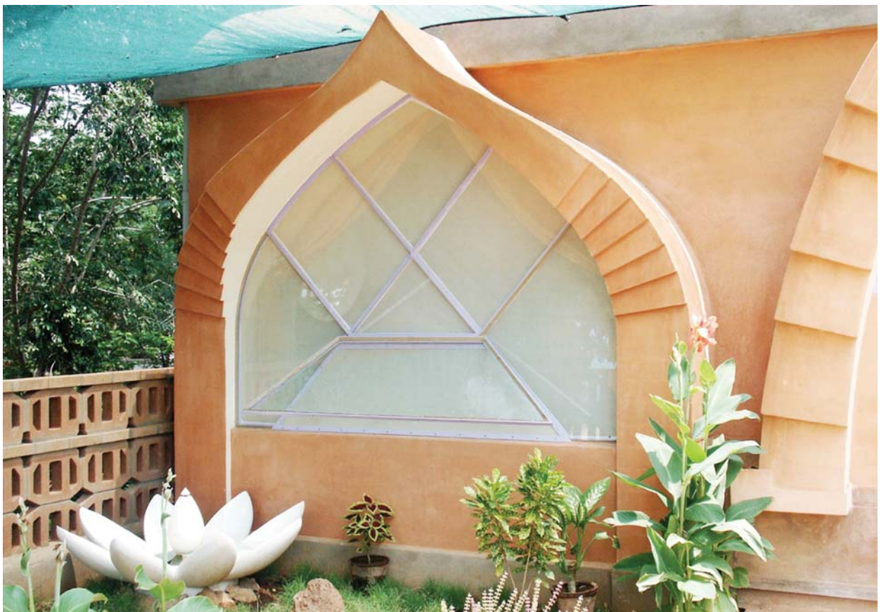
House at the Auroville Earth Institute
