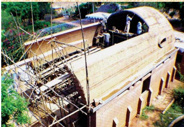
Building a semicircular vault with the Free Spanning technique - 6 m span, 11 m long
