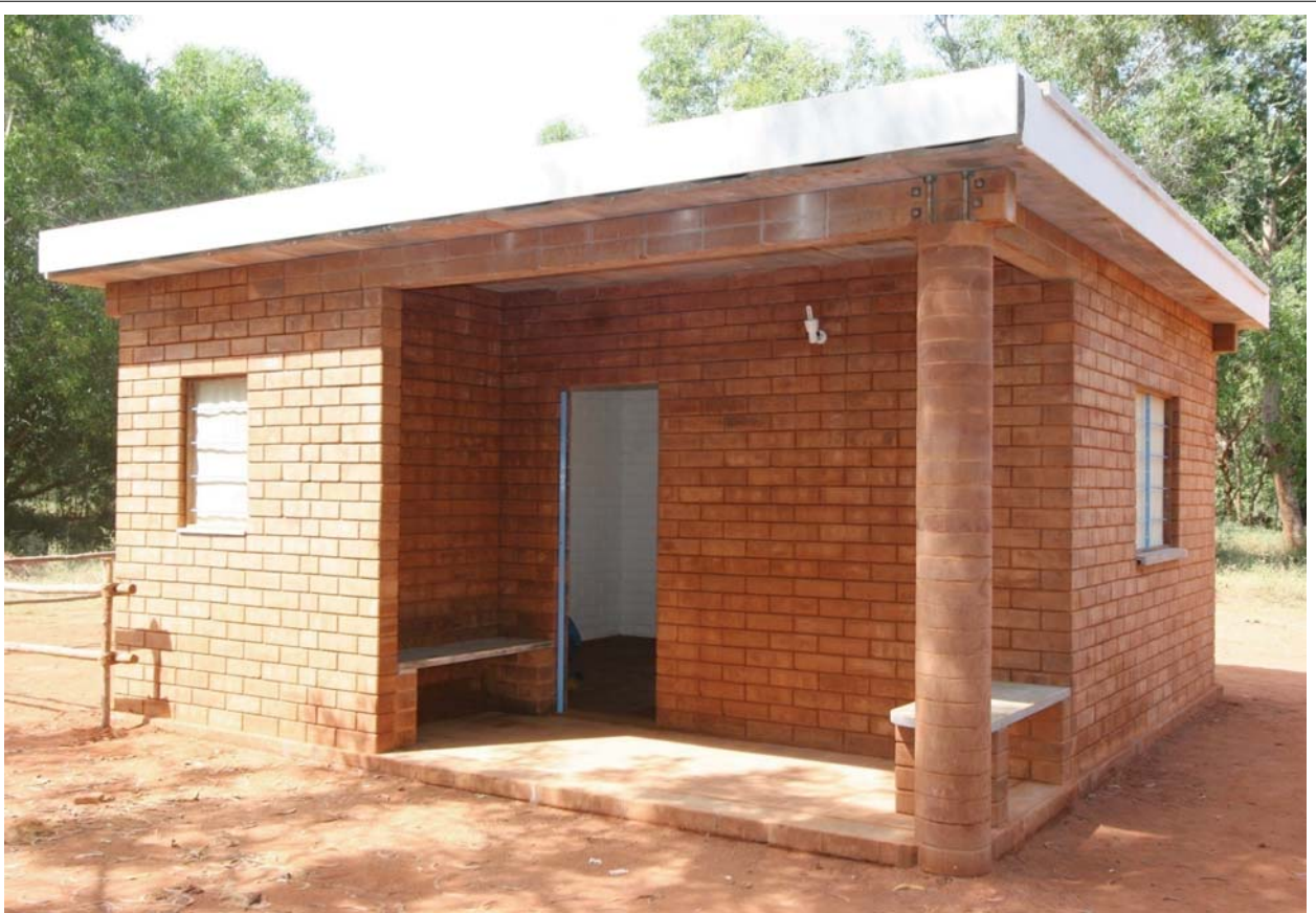
Auroville, Realization community – Moveable house, earthquake resistant, built in 64 h.
