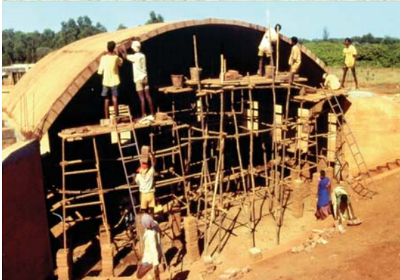
Deepanam School near Matrimandir - Stabilised rammed earth walls and CSEB vault, 10.35 m span -
