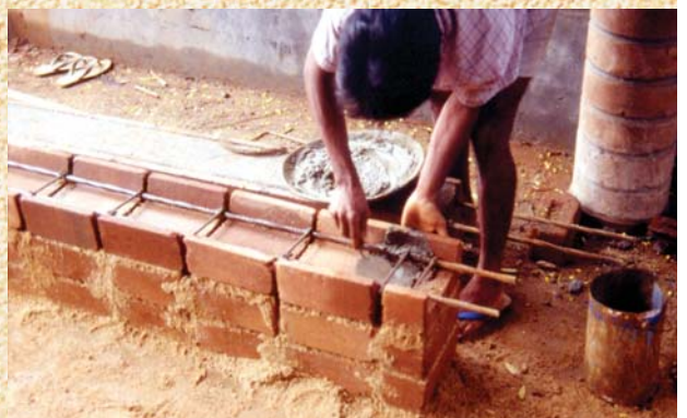
Composite beam triple height
