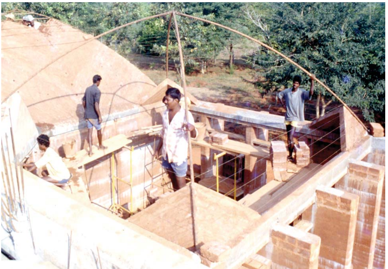
Building a cloister dome with the Nubian technique
