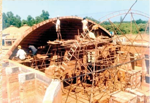
Deepanam School near Matrimandir - Stabilised rammed earth walls and CSEB vault, 10.35 m span -
