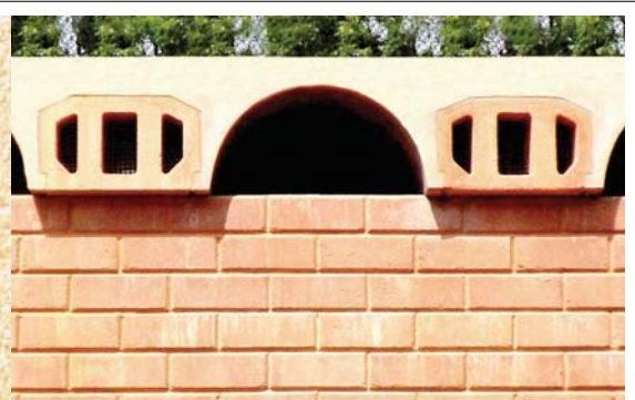
Hourdis blocks and ferrocement channels
